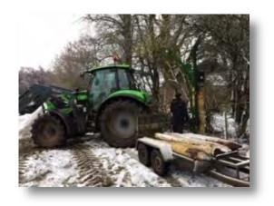
The contract was finally given to Gillan Fencing of Kirknewton. They cut back the hedgerow to allow for fence installation, removed all deadwood from North field boundary (which resulted in 10-15' of additional land gained over roughly 70m), installed 15 straining posts (some of which had to be dug by hand),
