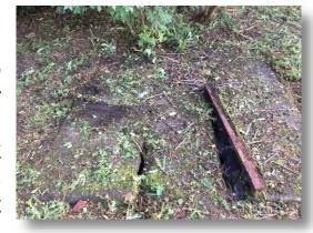
also damaged along the adjoining sides creating gaps that were unhealthy, dangerous and allowed rats to enter the tank.
